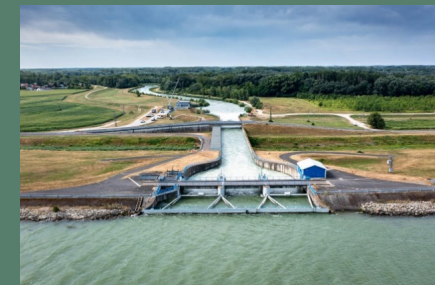
Picture 4: Artificial inlet object from the canal to the side-arm system (author: VVB, 2023)
