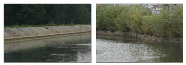
Asphalt bank protection before revitalisation and revitalised bank protection
